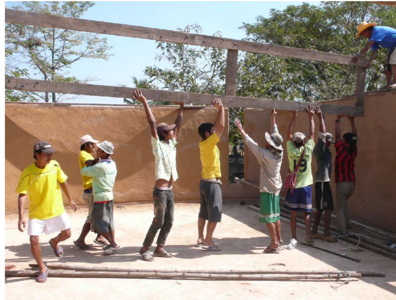
top right: Lifting up the frame
